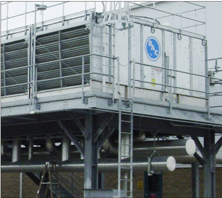
Bottom Inlet EASY CONNECT® Piping Arrangement Installation
