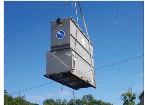
Single Piece Lift of a VTO Cooling Tower
