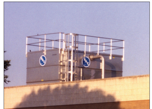
Handrail and Ladder Package
