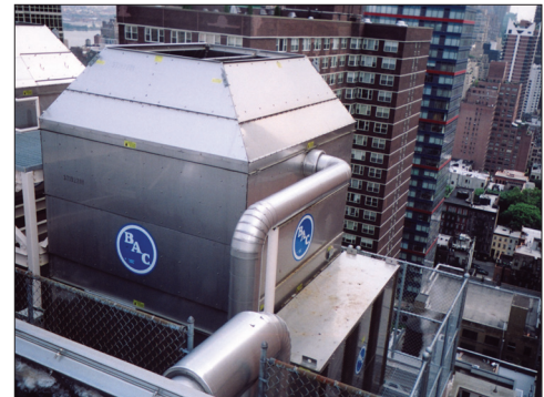
Unit with Intake and Discharge Sound Attenuation
