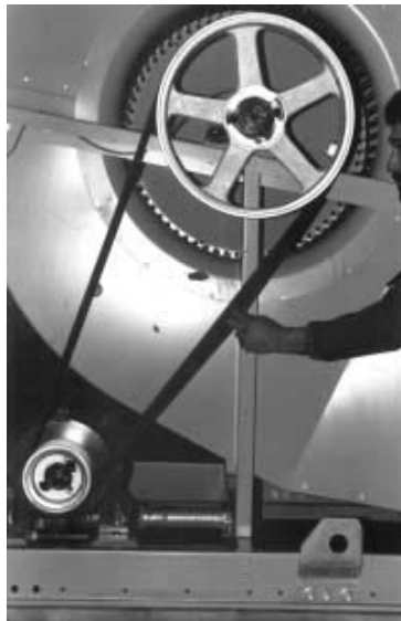
Figure 11. Fan Belt Adjustment
