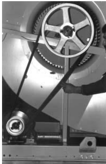
Figure 11. Fan Belt Adjustment
