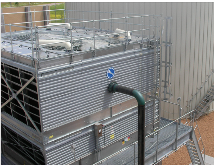
Seismic/Wind Upgraded Structure with Fiberglass Reinforced (FRP) Casing Panels
