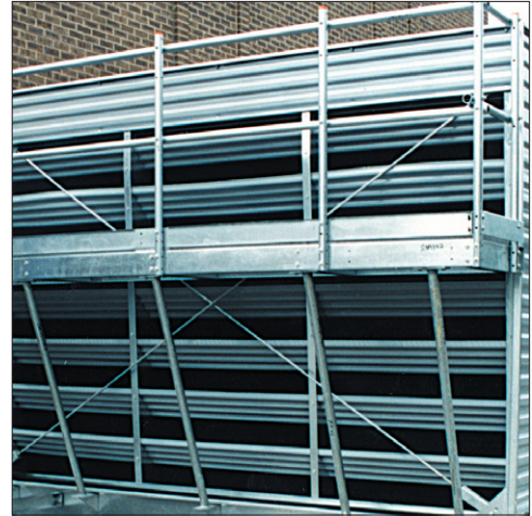
External Ladder and Platform
