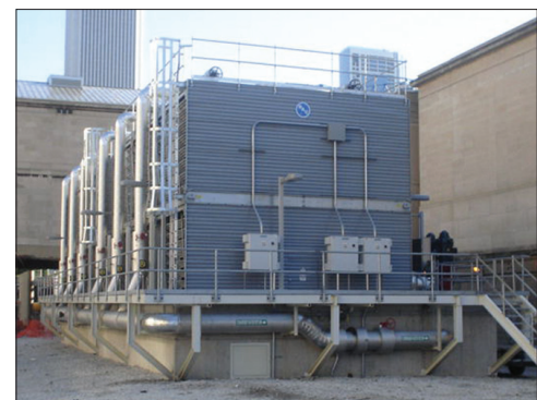
Flexible Piping Arrangement
