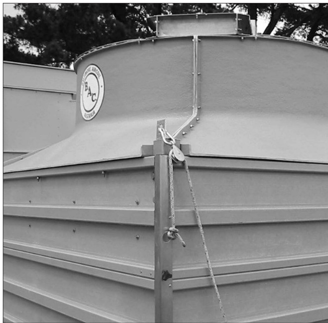
Figure 8. Access Door Anchor Points
