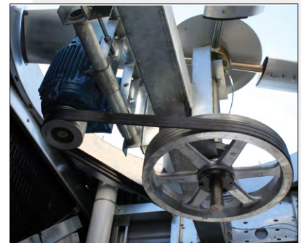
Figure 2. BALTIDRIVE® Power Train
