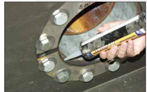
Figure 17. Caulk Exposed Galvanized Steel
