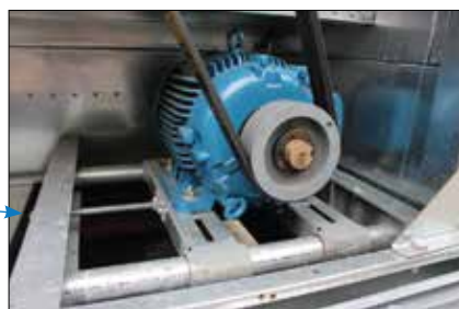
Figure 4. Motor Adjusting Screw
