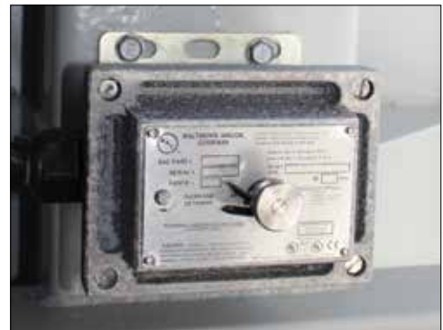
Vibration Cutoff Switch
