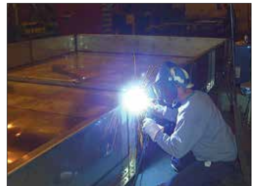
Welded Stainless Steel Basin
