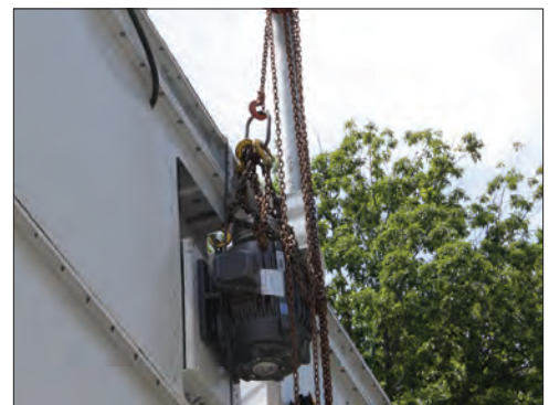
Motor Removal System
