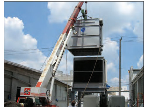
Modular Design Simplifies Rigging
