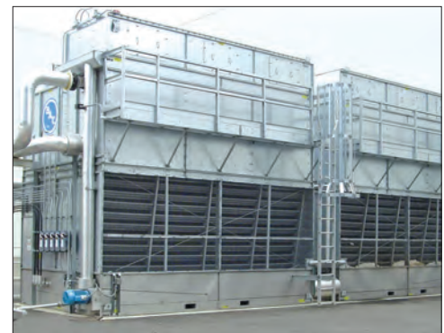
PCD Hood Installation
