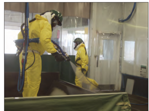
Application of TriArmor® Corrosion Protection System
