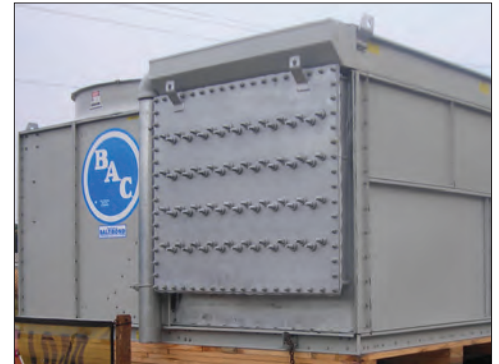
Straight-Through Cleanable Coil
