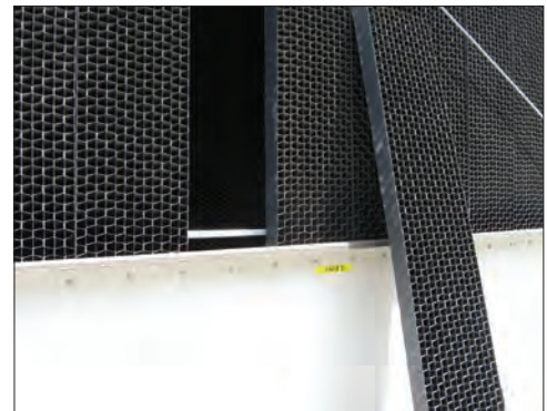
Combined Inlet Shields
