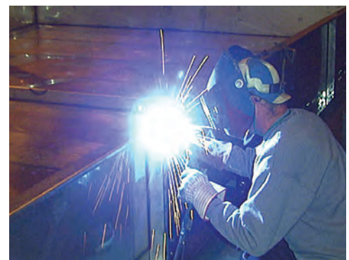
Welded Stainless Steel Basin
