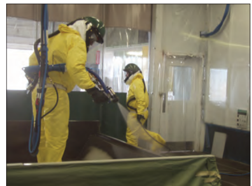
Application of TriArmor® Corrosion Protection System
