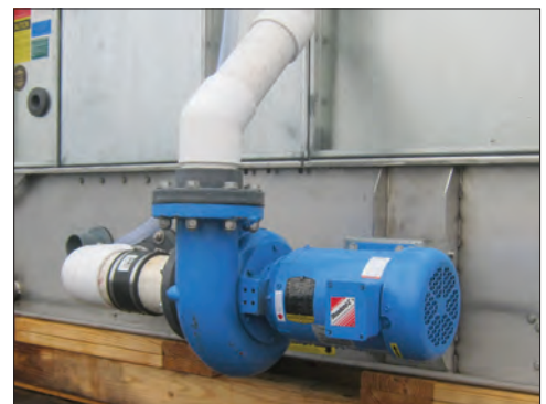
Standard Spray Water Pump
