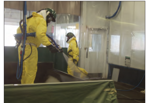
Application of TriArmor® Corrosion Protection System
