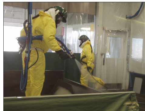
Factory Application of TriArmor® Corrosion Protection System
