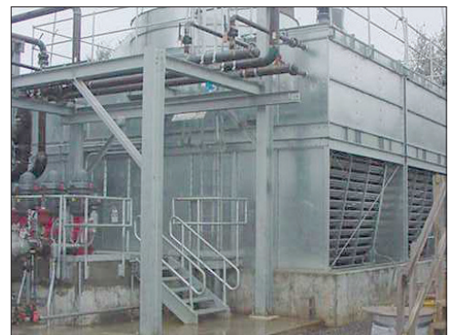
Basinless Unit Construction
