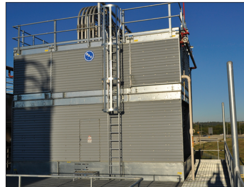
Standard Construction Installation
