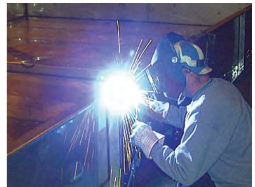
Welded Stainless Steel Cold Water Basin
