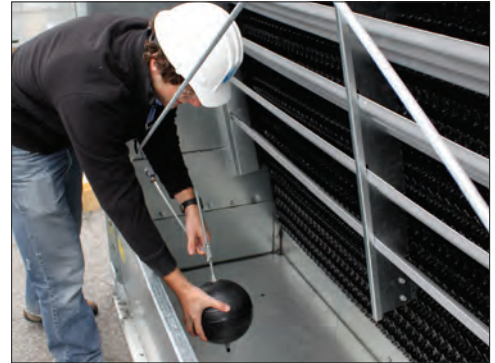
Mechanical Water Level Control
