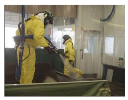
Application of TriArmor® Corrosion Protection System
